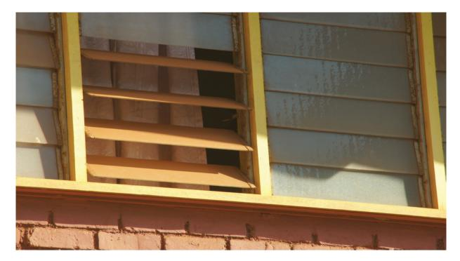
Figure 4: Red dust deposited on window of quarter next to Kuantan Port
