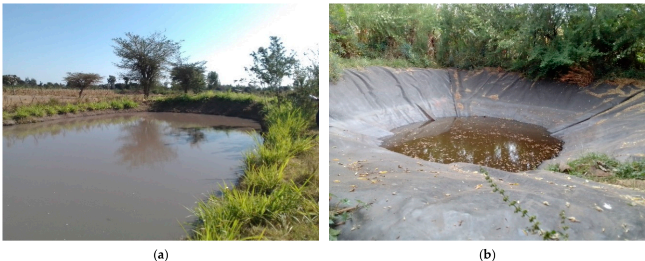
Figure 9. Typical water harvesting ponds: (a) large and unlined, (b) small and lined.
