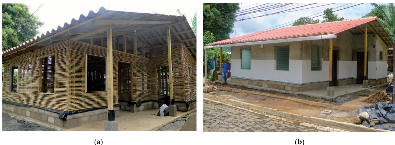
Figure 2. Photographs showing prototypes built in 2012 of the CBSW system developed for El Salvador [9,14]: (a) prior to plastering with render; (b) completed house.
