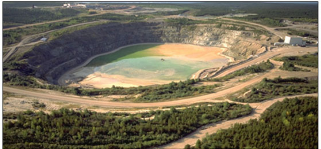
Figure 15. Rabbit Lake in-pit disposal of mine tailings—Tailings beach overview.
