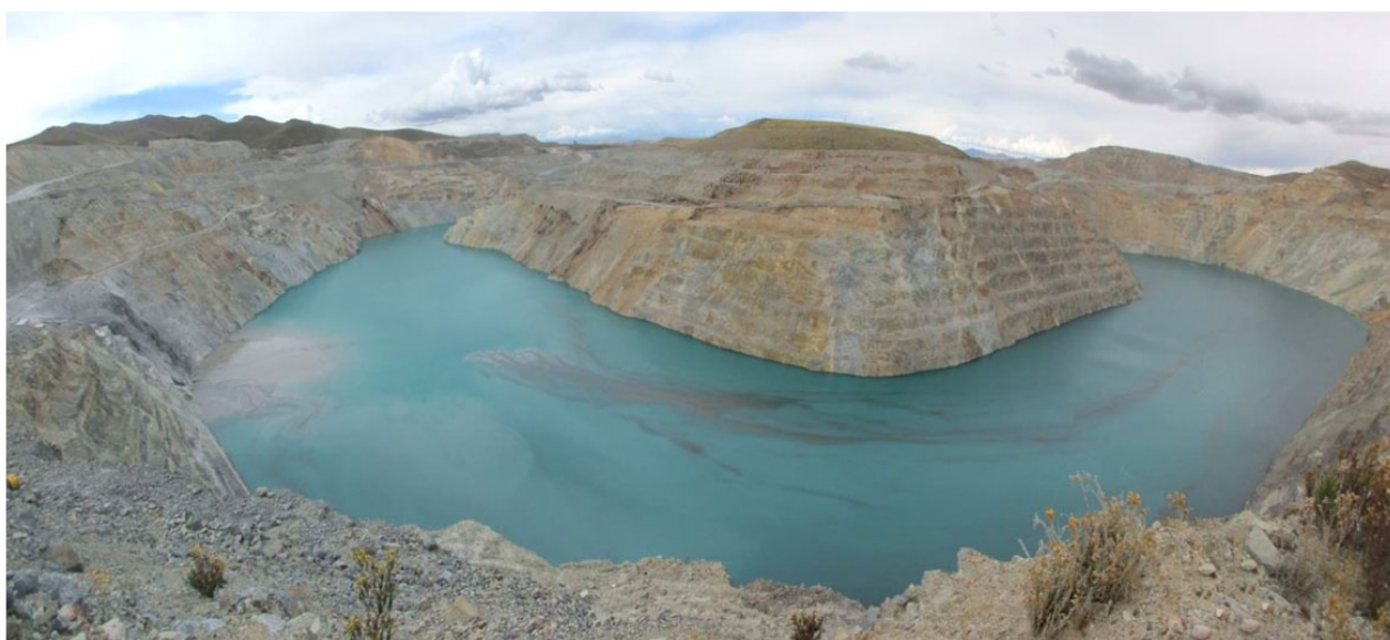
Figure 14. In-pit disposal of mine tailings and water management at old Tintaya open-pit mine.
