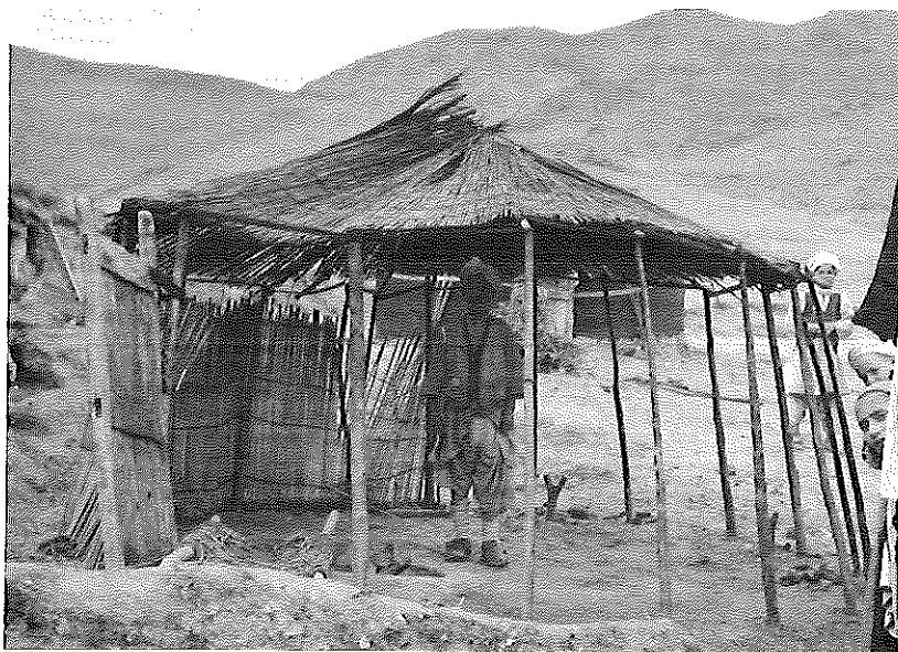
Fig. 9. The framework in a Firôzkôhi chapari . To the upper end of every side stick, embedded in the ground, is bound a straight roof stick. These are then bound together in the centre to form a conical roof. The roof is covered with willow mats ( chigh ), and the side cover is either of felt or black woollen cloth ( palâs ) plus chigh . From the village Delma, ca. 10 km E. of Chisht on the Harî Rûd. 30/11-1954.
